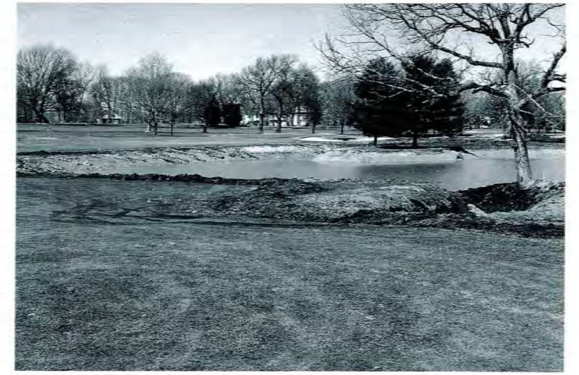
Wannamoisett's Pond at #14 Under Construction.
